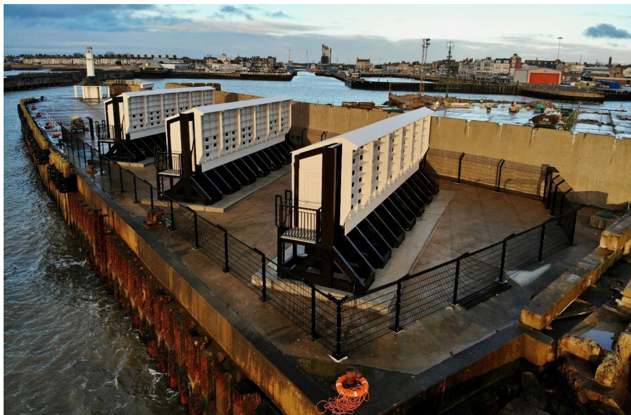
Figure 4: Photo of the three wall structures as constructed at the Port of Lowestoft (February 2023)
